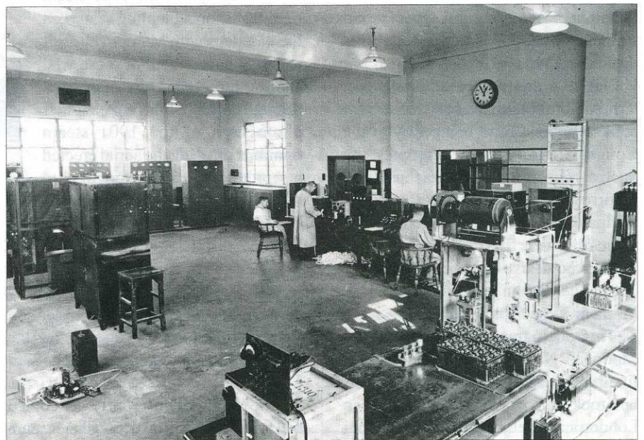
Photo 5 - In 1937 a new transmitter station was opened at West Wickham, Kent, about 15 miles from New Scotland Yard. The transmitters were remotely keyed from the wireless operators' position at NSY via a VF system (see Photo 4).
